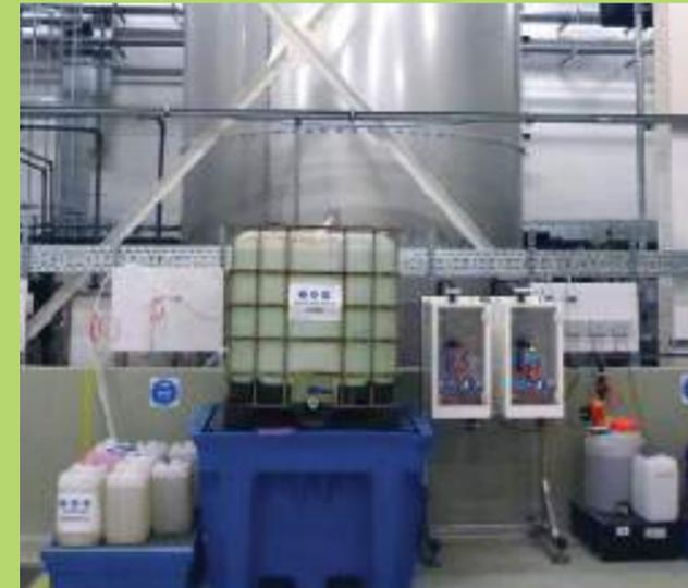
Figure 12.3 Physical-chemical treatment with chemicals (left) and ozone (right)
