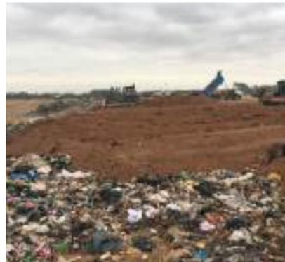
where cover soil is in short supply, or where artificial cover methods such as tarpaulins are being used) this may not be enough on its own to provide effective litter control and additional measures to control litter may be needed (see the Guideline for Litter Control).
