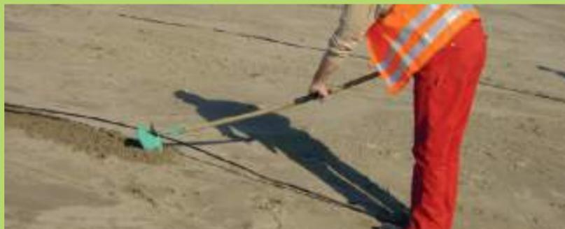
**Figure 19.8.** Installing cables and electrodes of a leak detection system.
