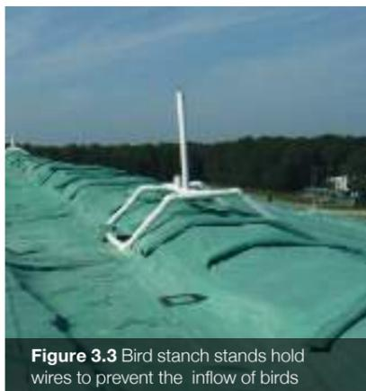
Figure 3.3 Bird stanch stands hold wires to prevent the inflow of birds
