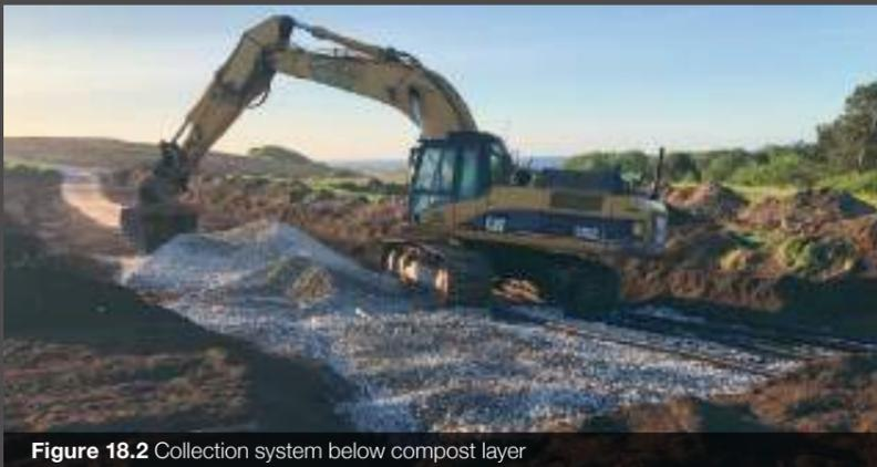
Figure 18.2 Collection system below compost layer
