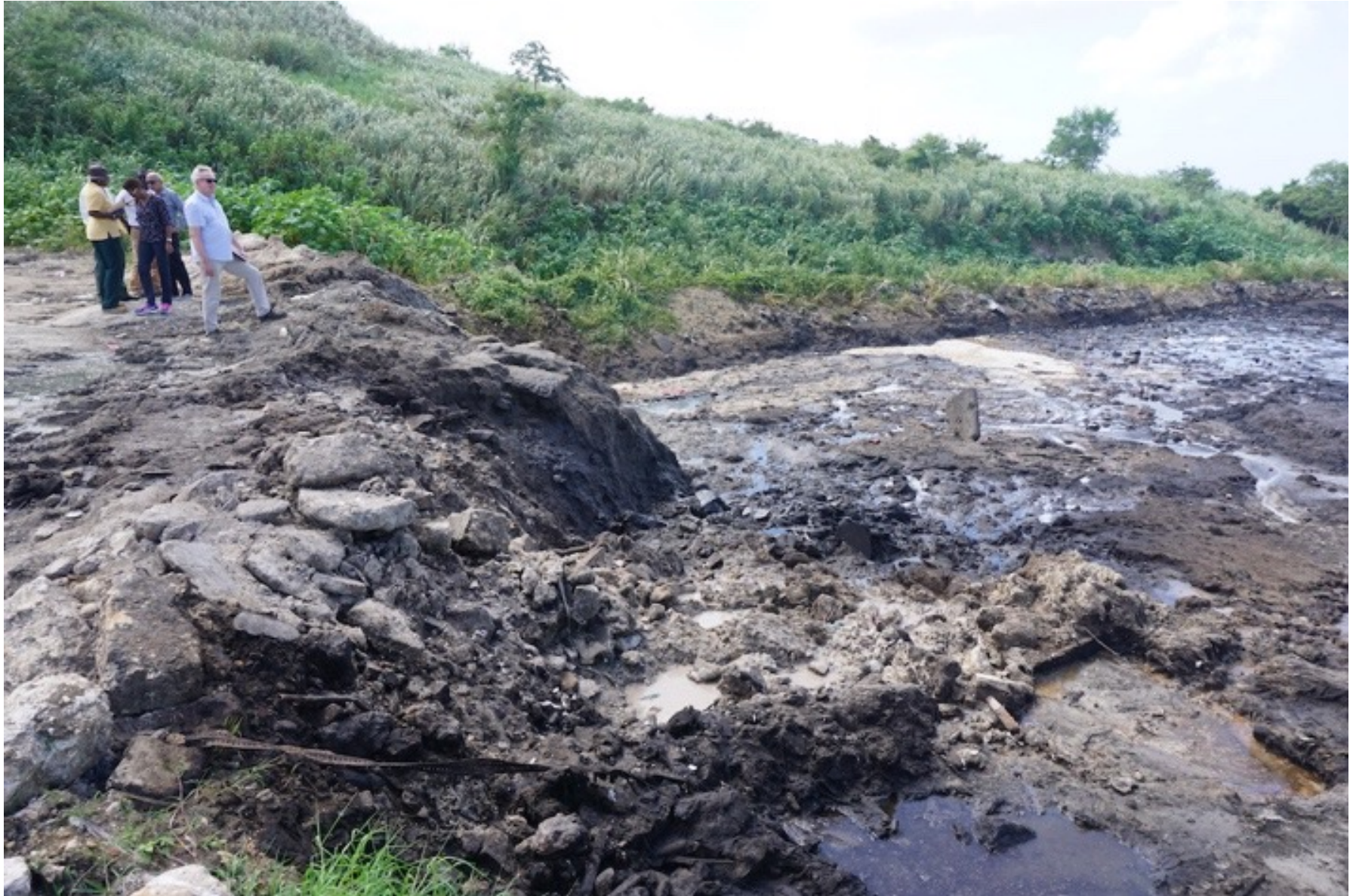
Unlined liquid waste pond at Mangrove Pond Landfill area, Barbados
