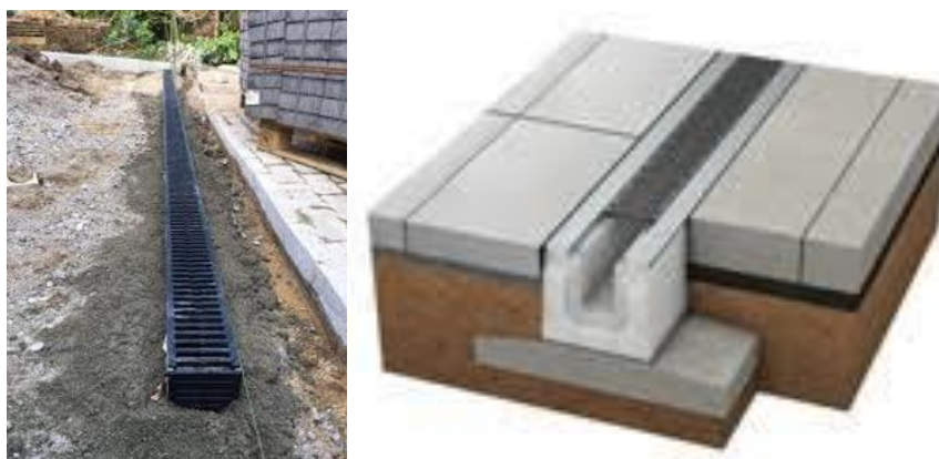
Figure 8: Example of traversable gutter to be installed along the front side of the HWISF
