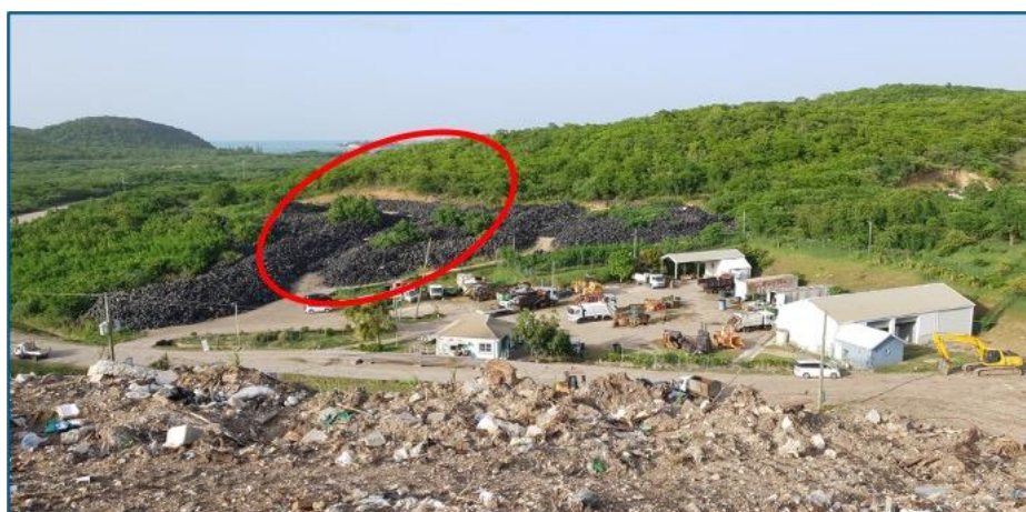
Figure 10: Proposed location of the Hazardous Waste Interim Storage Facility, currently used for storage of waste vehicle tyres.
