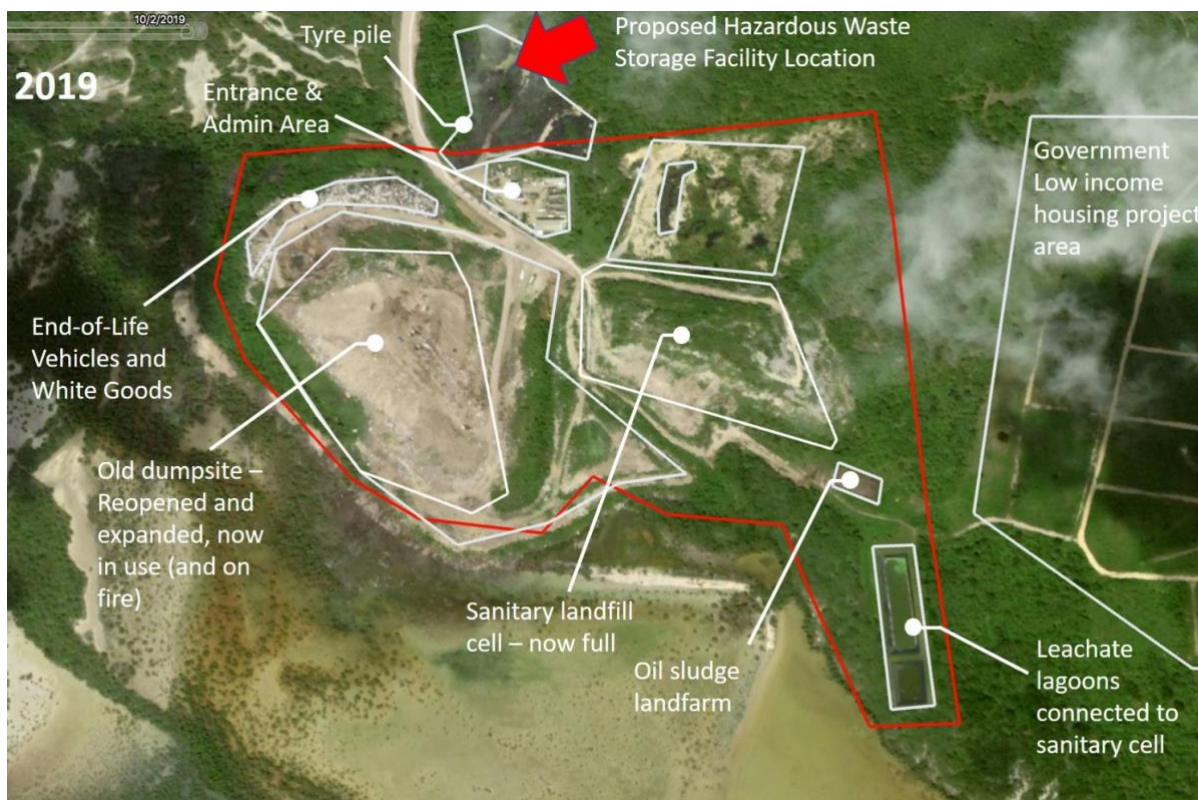
Figure 5: Proposed location of Hazardous Waste Storage Facility in relation to Cooks Landfill site infrastructure
