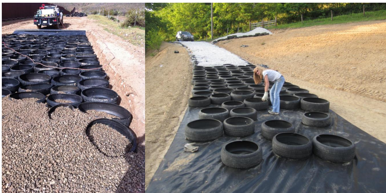
Figure 13: Gravel fill of tyre cylinder geogrid once in place http://www.mechanicalconcrete.com/county-takes-green-approach-to-roadbuilding/ .
