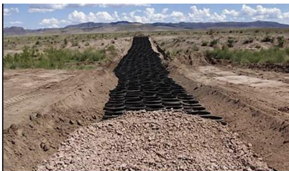
Figure 14: Gravel Road construction http://www.mechanicalconcrete.com/county-takes-green-approach-to-roadbuilding/
