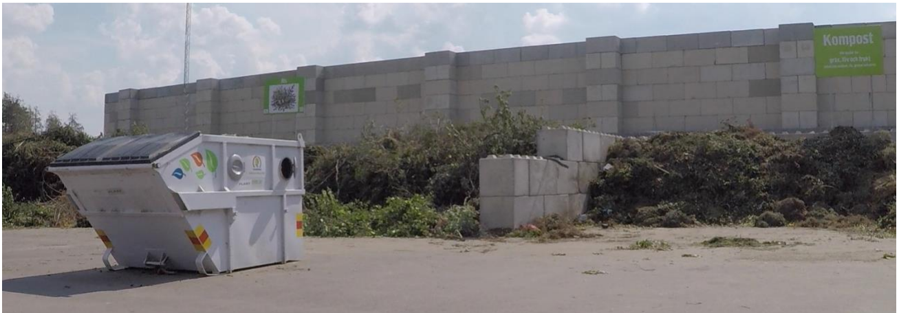
Figure 9: Green waste drop off with container for bags and other foreign objects, also divider wall to separate tree cuttings from smaller grass cutting and pre-shredded material - Eskilstuna landfill in Sweden
