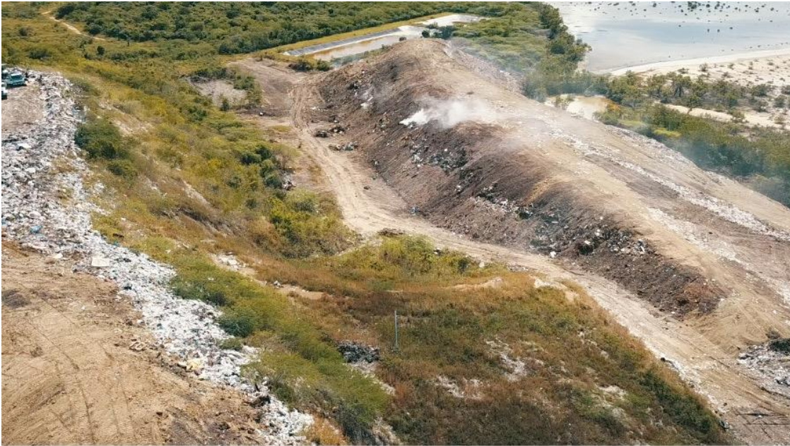
Cooks landfill on fire with smoke, including unintentional Persistent Organic Pollutant (uPOPs), emissions visible along the edge of the landfilled waste mass.
