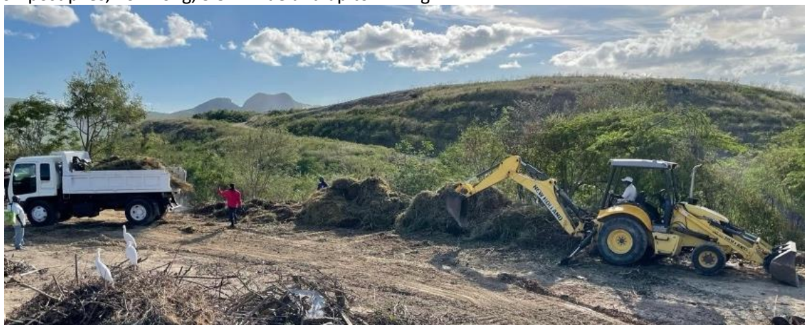
Material will be layered with alternating layers of nitrogen rich greens, and carbon rich wood chips. Each layer must be watered down heavily as the pile is constructed, water pumps are provided.
